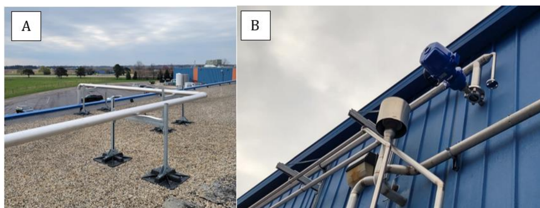
Figure 3. Installed roof piping A – roof at IB3A side, B – IB1a end with isolation valve.
